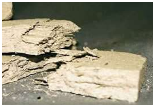
Pieces of Asbestos Insulating Board (AIB)
