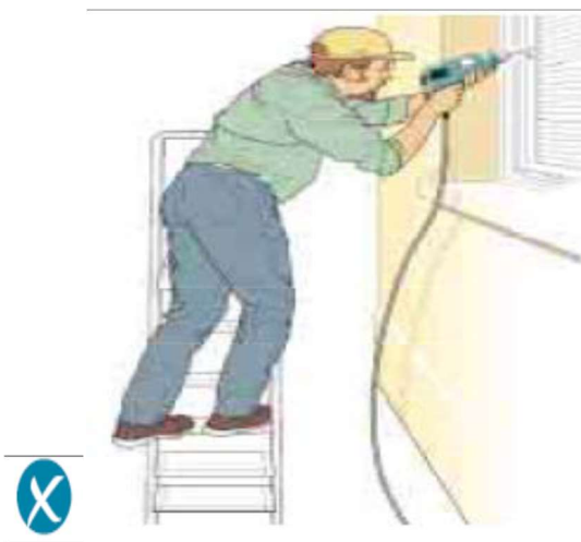
Incorrect – steps side on to work activity
