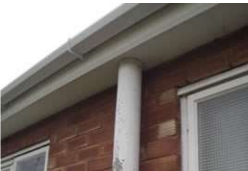
Asbestos cement drainage pipe (downpipe)
